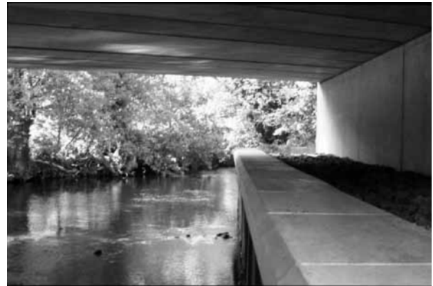
Figures 68 and 69. Large culvert with shelves to allow animals to safely cross the road (Photo: Grogan et al., 2001)
